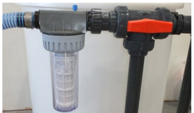
Heavy duty filter and 3-way valve
